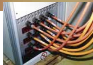
Connection of the measuring cables to the system
