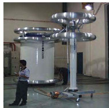
System with 300 kV test transformer and HV divider
